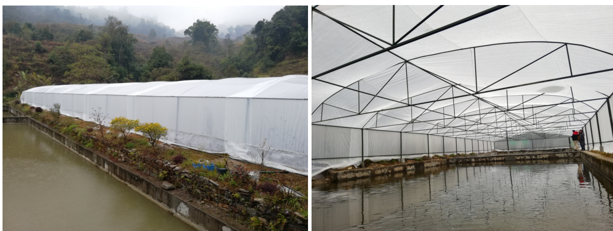
Figure 4: Construction of 160 ft*40 ft greenhouse /plastic tunnel at Rupa Fish Hatchery, Chaur.
